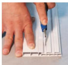
**Option 1B:** Cut to have the height 60 mm.
