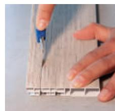
2. Cut the skirting on the front side at the cut previously made on the back;
